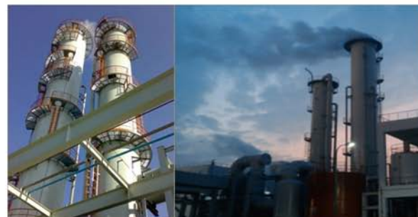
100 kt/a CO 2 capture demonstration in Huaneng Shanghai Shidongkou Power Plant
